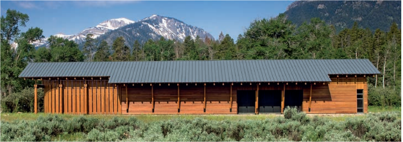
Laurance Rockefeller Preserve, Grand Teton National Park, Wyoming, USA LEED™ Platinum Certified – Carney Logan Burke Architects, Jackson, WY, USA Application: Double Standing Seam Panels, RHEINZINK-prePATINA graphite-grey
