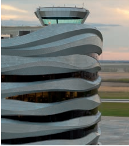
Edmonton International Airport, Edmonton, Alberta, Canada – LEED™ Silver DIALOG Architects, Edmonton, AB, Canada Application: Flat Lock Tiles, RHEINZINK-prePATINA blue-grey
