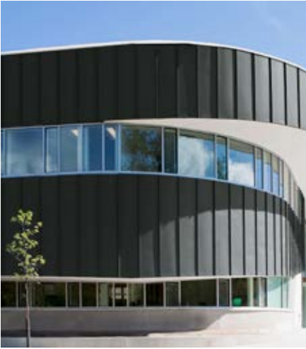
Simcoe County Admin Building, Midhurst, ON, Canada – LEED™ Gold Teeple Architects, Toronto, ON, Canada, Application: Vertical Reveal Panels, RHEINZINK-prePATINA graphite-grey
