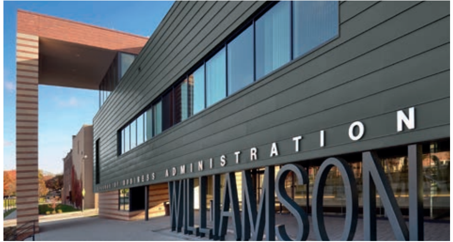
Williamson College of Business Administration, Youngstown State University, Youngstown, OH LEED™ Gold – Perkins+Will, Minneapolis, MN and Strollo Architects, Youngstown, OH Application: Angled Standing Seam Panels, RHEINZINK-prePATINA graphite-grey
